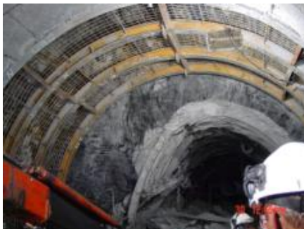
Rehabilitation of the tunnel profile after large convergences Yacambu – Quibor - Venezuela
