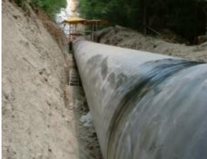
Replacement of the Peuffeyre penstock Switzerland
