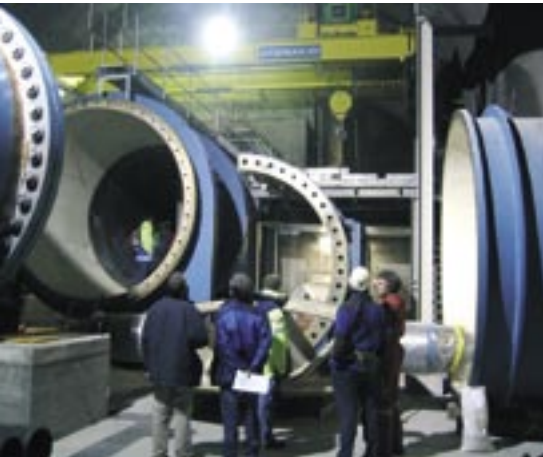
Cleuson-Dixence Scheme, rehabilitation of the underground penstock, Switzerland
