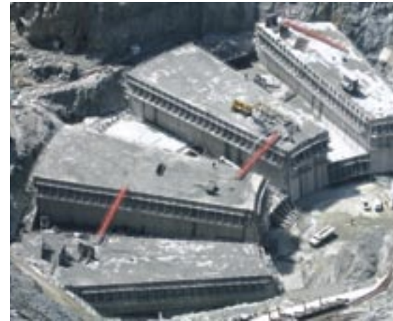
Deriner Arch Dam, first concrete lifts, Turkey
