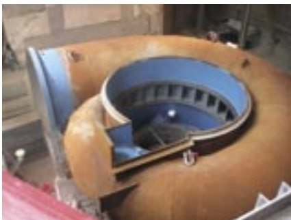
Rehabilitation works at the Hauterive HPP, Switzerland
