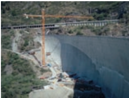
Strengthening works of Les Toules Dam, Switzerland
