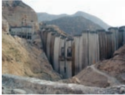
Karun IV Arch Dam, Iran
