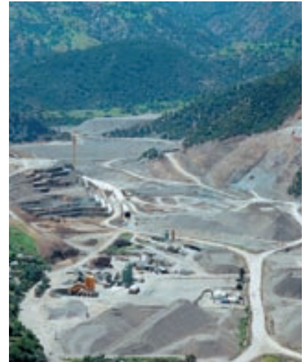
Kef Eddir Dam, Algeria
