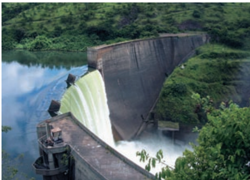
Rehabilitation and heightening of Cambambe Arch Dam, Angola
