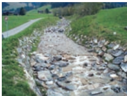
Block ramp on the Flumy River, Switzerland
