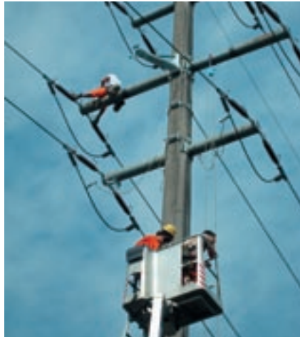
Volta-Joule and Volta-Ampere transmission line Connection of 65 kV cables' terminations, Switzerland
