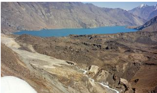
Figure 1. Aerial view of Usoy dam. The RBS is in the background.
