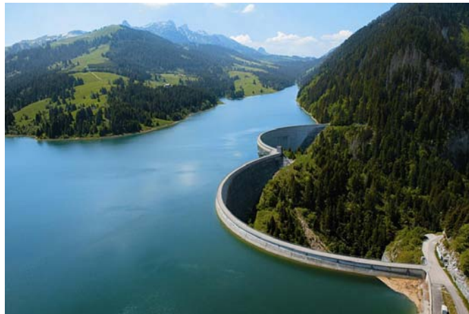
Figure 1: Hongrin dams (north 125 m / south 95 m high)
