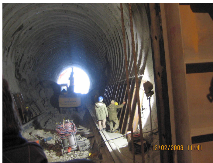
Figure 9. Overflow spillway on the right bank: photos made during construction.
