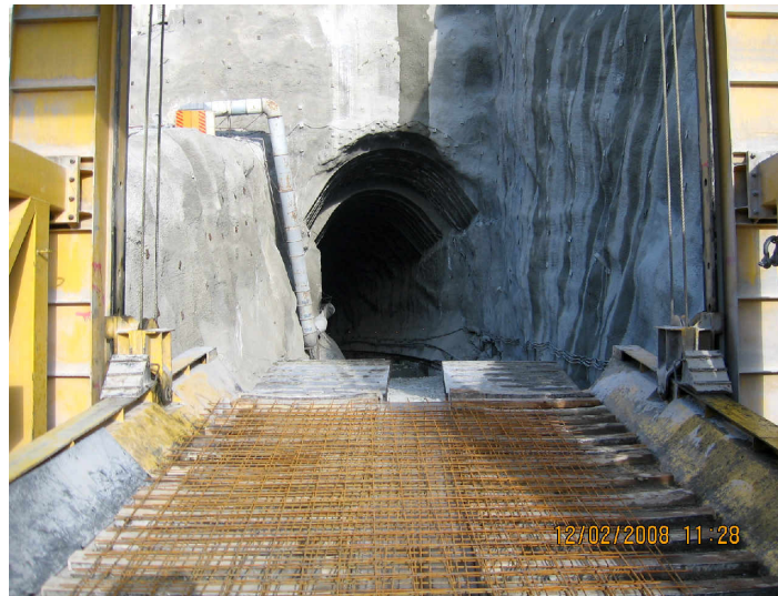
Figure 8. Rock support of the overflow spillway on the right bank.
