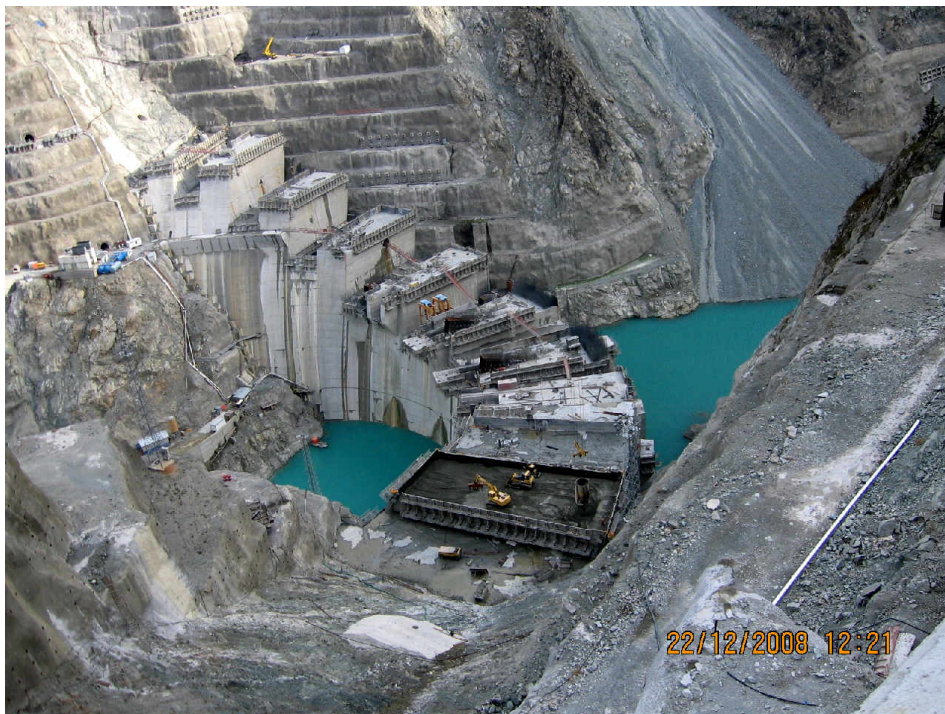
Figure 2. Deriner HEPP, state of construction in December 2008.
