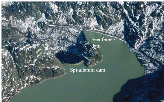
Figure 4: Picture with Seeuferegg gravity dam and Spitallamm arch-gravity dam
