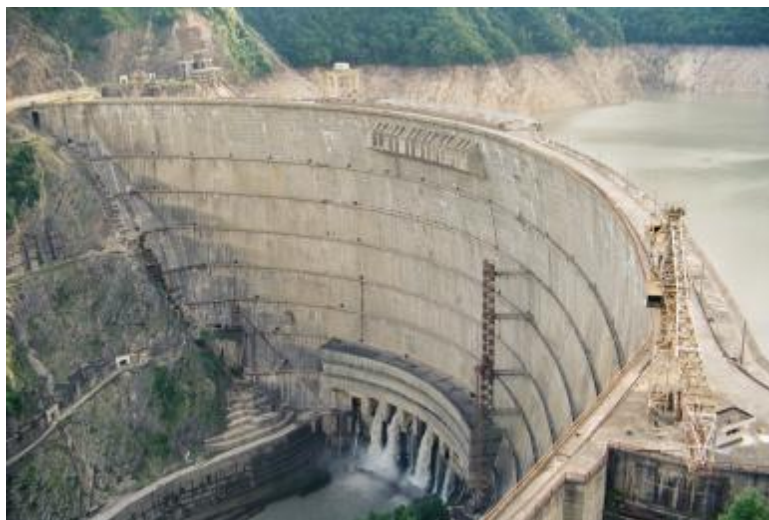
Figure 4. Enguri Arch Dam in Georgia, 271.5 m high
