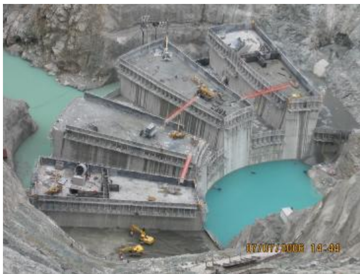
Figure 3. Deriner arch dam (Turkey), 253 m high, under construction
