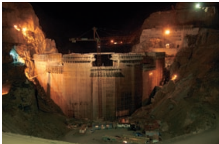
Barrage de Shahryar (ex Ostour) - Iran
