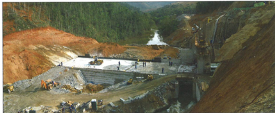
The Picada RCC dam under construction, view from downstream. Image: Stucky.
