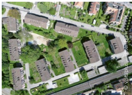
Top: Aerial view of the major job site in the Swiss capital of Bern. Bottom: The site was previously occupied by small-scale apartment buildings.
