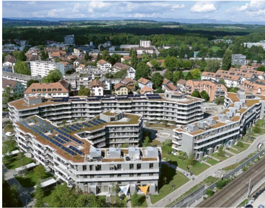
Rooftop solar collectors – the Stöckacker Süd estate is run entirely on alternative energy.
