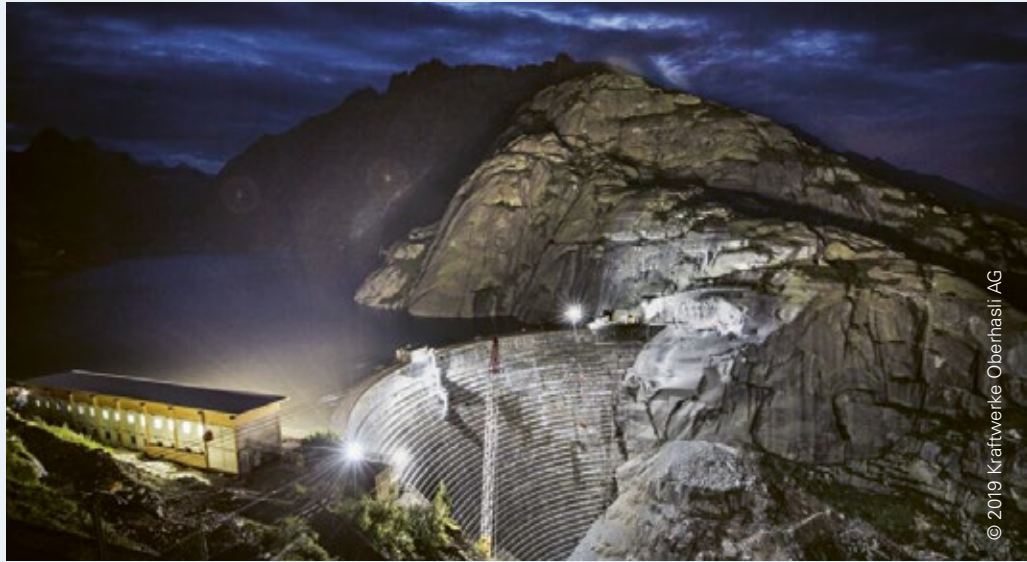
Job site with existing dam at an altitude of nearly 1,900m.
