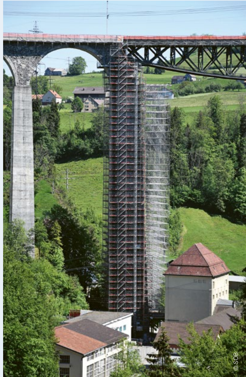
Work location at a height of nearly 100 m.
