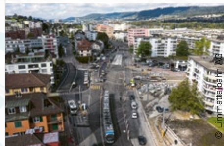
... and the journey now continues to Schlieren on newly laid track.
