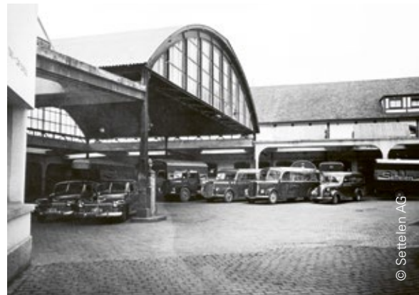
As early as the start of the last century, the prestigious steel and glass barrel-vault roof provided a sheltered courtyard area.
