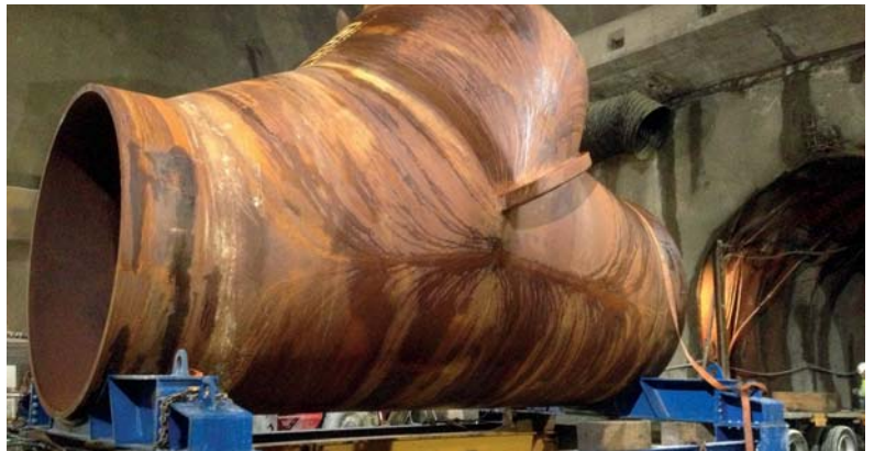
Penstock manifold (Hongrin-Léman Pumped Storage Scheme), Switzerland
