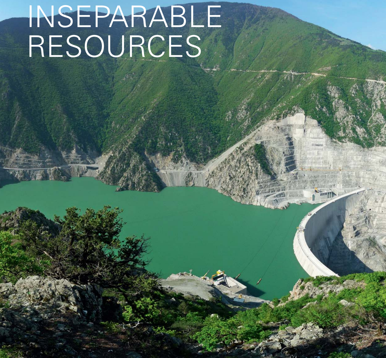
Deriner Dam and Hydropower Plant, Turkey
