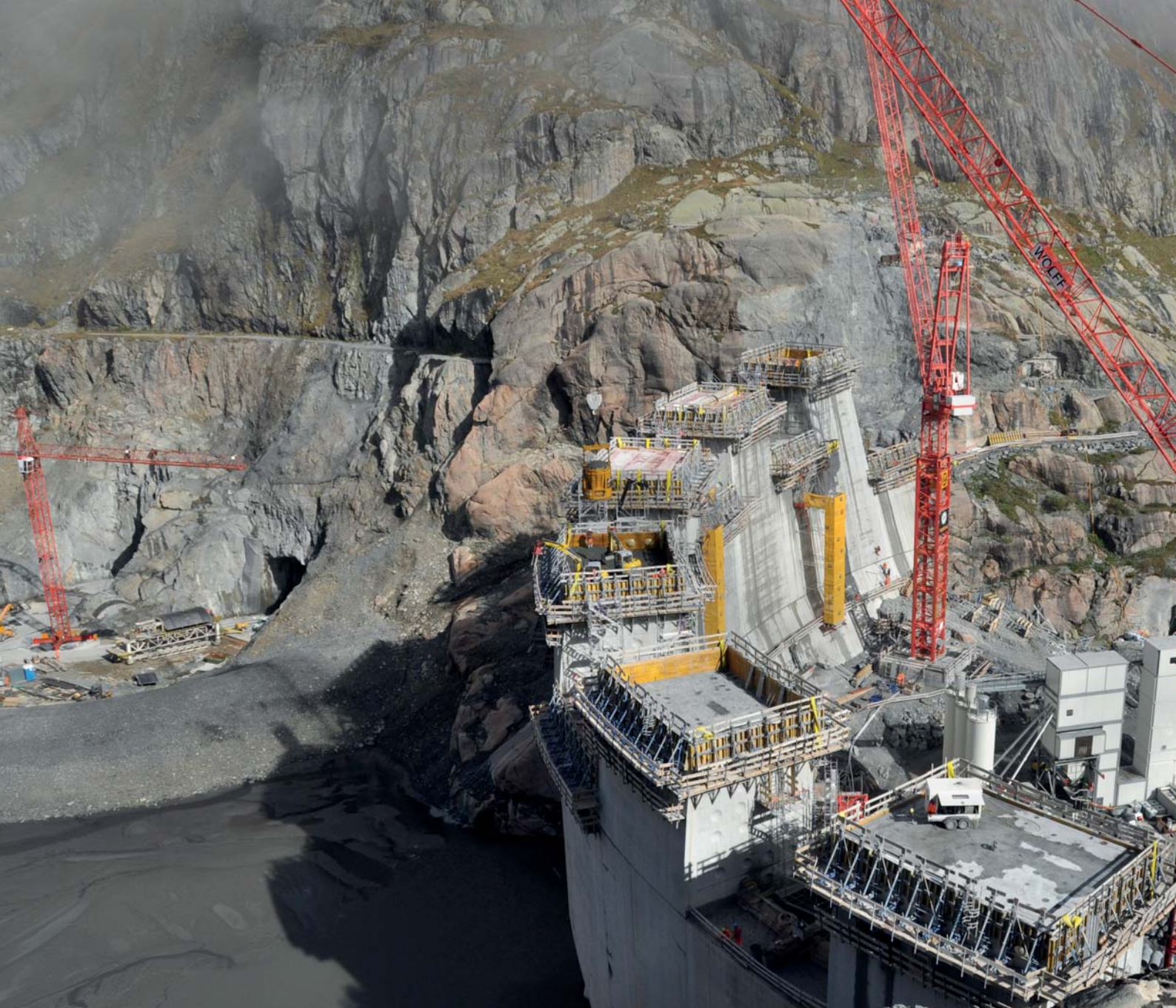
Heightening of Vieux Emosson Arch Dam, Switzerland
