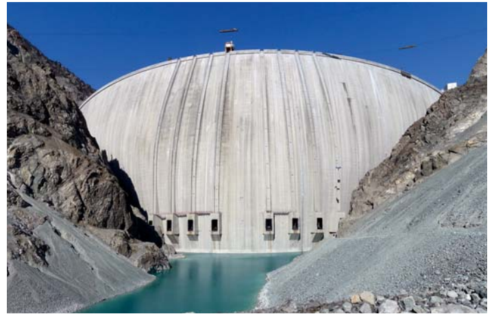
Deriner Arch Dam, Turkey
