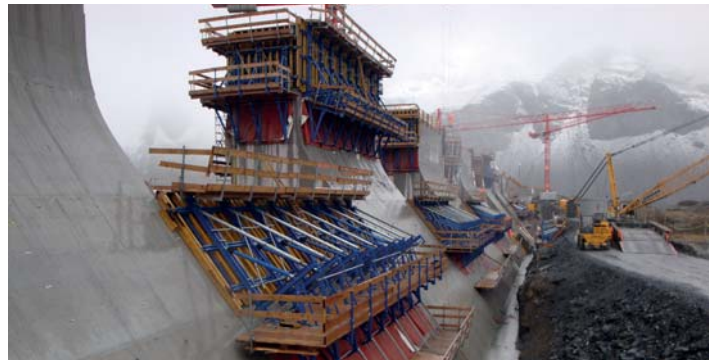
Muttsee gravity dam, Switzerland
