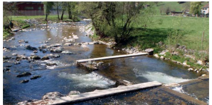
Fish Ladder Aubonne, Switzerland
