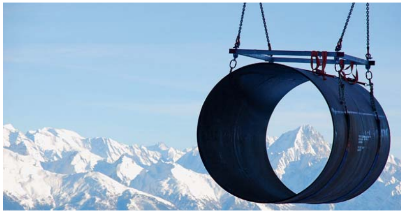
Replacement of the Penstock, Cleuson-Dixence hydropower plant, Switzerland
