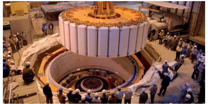
Karun IV powerhouse, Iran
