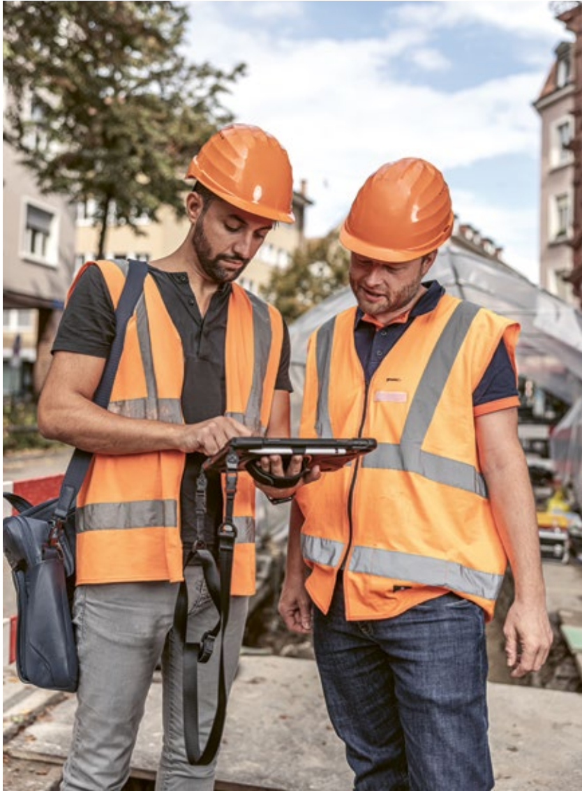
Our civil engineering site supervisors Danilo Rizzo and Reto Hügi are on site practically every day to monitor the progress of the works using BIM to Field. Visible in the background is the tent protecting the archaeological excavations.
