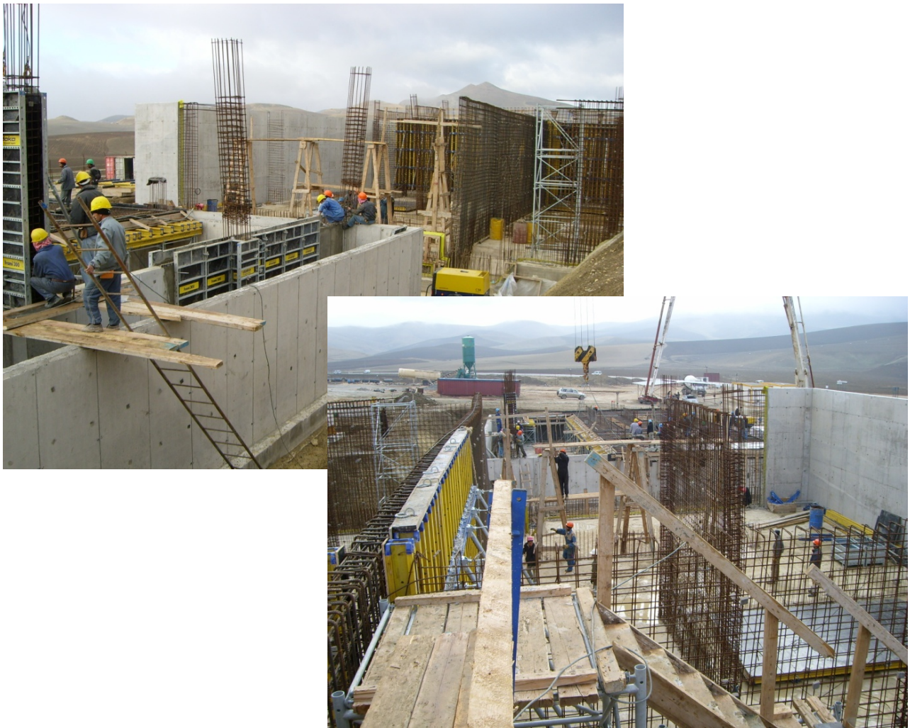
Construction of a pumping station
